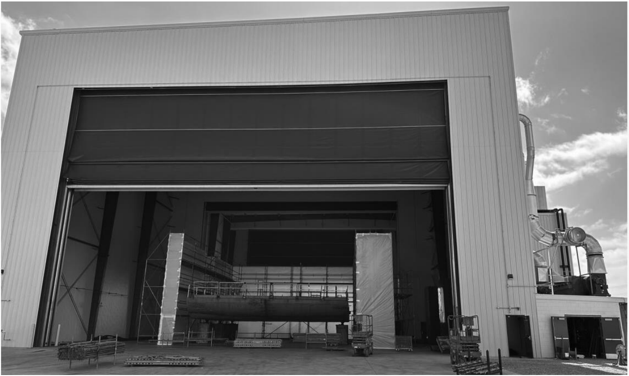
Fig. 6, Blast and Paint Booth with Middle Door View 2
