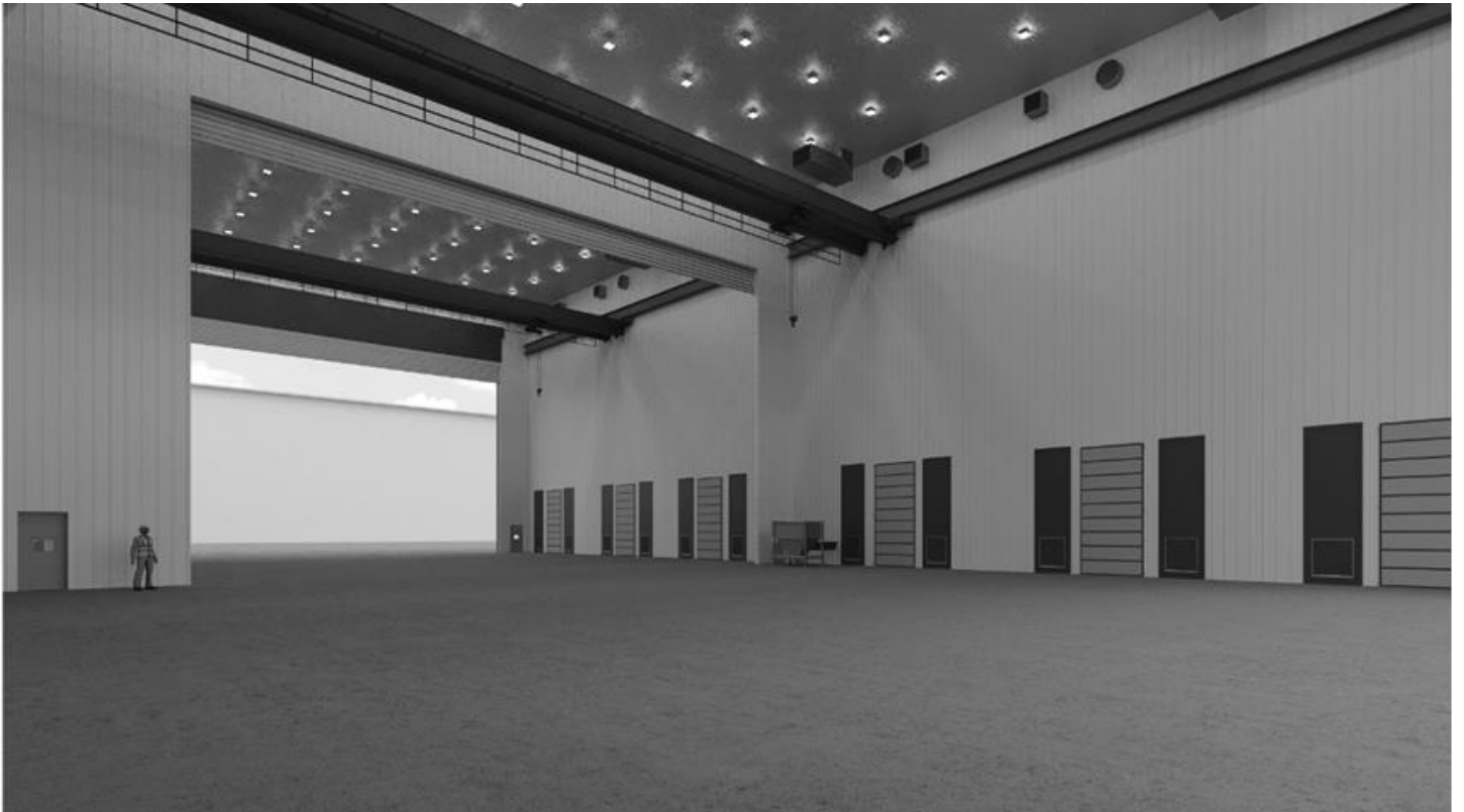
Fig. 8, Blast and Paint Booth with Middle Door and Overhead Crane
